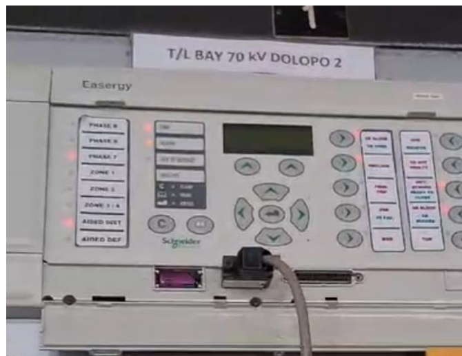
Gambar 21. Relay Distance Gardu Induk Ponorogo.
