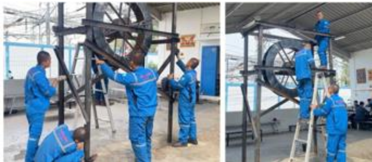
Gambar 12. Proses Assembly PLTMH.
