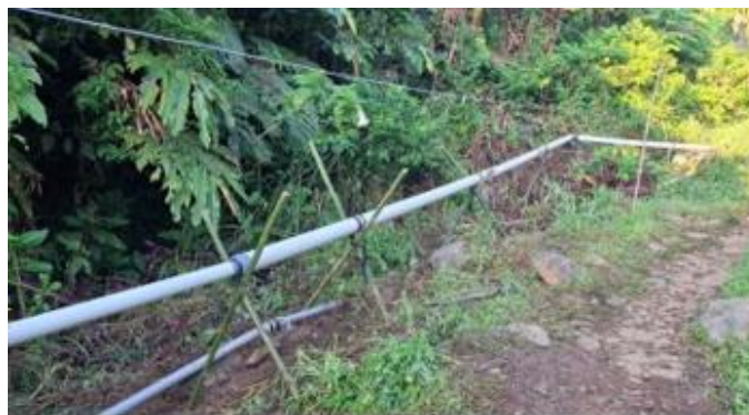
Gambar 13. Instalasi Pipa Pesat (Penstock).
