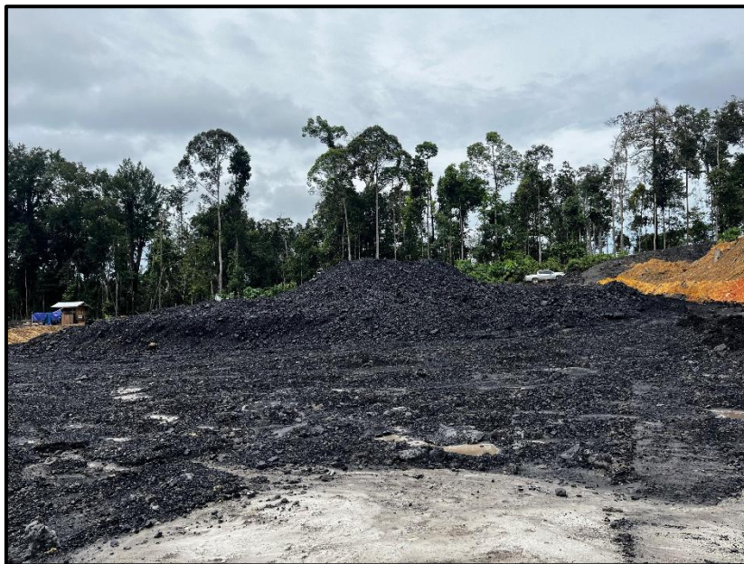
Gambar 2 Lantai dasar stockpile baru.
