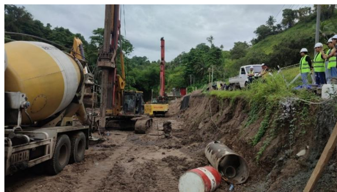
Gambar 1. Pengecoran Bore Pile .
