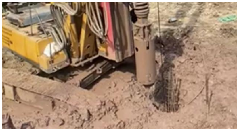
Gambar 5. Mata Bor revolving cutter bit .
