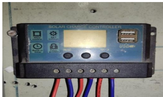
Gambar 10. Instalasi Solar Charger controller
