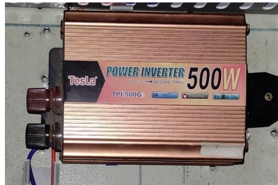
Gambar 11. Instalasi Inverter 500Watt
