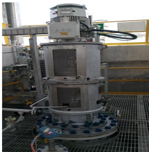
Gambar 1. Konfigurasi struktur closed drain pump
