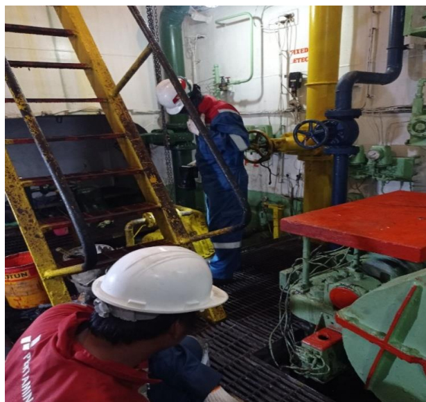
Gambar 3. Pengecekan Got Pump Room . Sumber: Penulis (2024)
