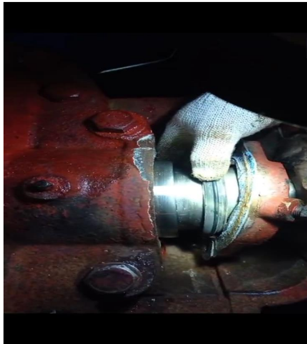
Gambar 2. Kebocoran Mechanical Seal
